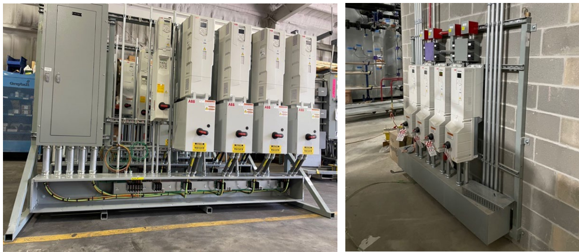
Figure 10: Prefabricated rack of VFDs (left) in the shop and (right) installed at sight
